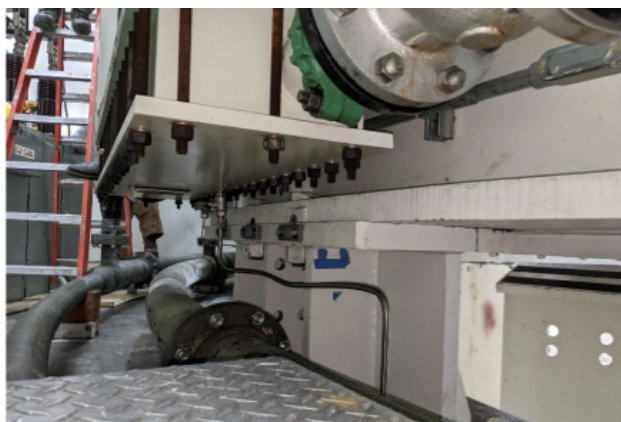
Fig 4 - Stator sole plate
