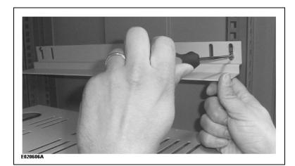
Install side mounting brackets and adjust at the correct height.
