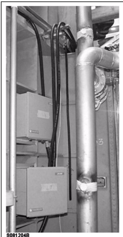
Figure 11 : Suitable location for a protection box
