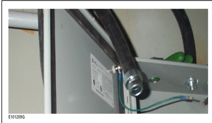
Figure 19 : Flexible conduit connection to enclosure
