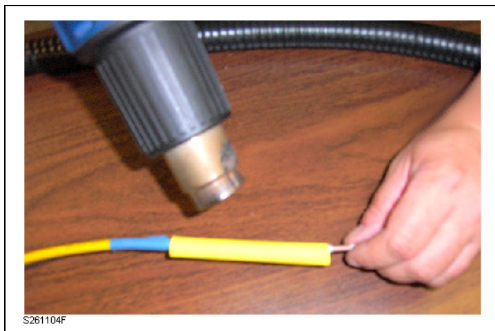
Figure 12 : Heating the heat-shrinkable tubing
