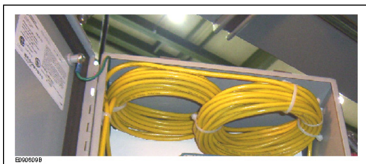
Figure 22 : Excess cable stored in enclosure
