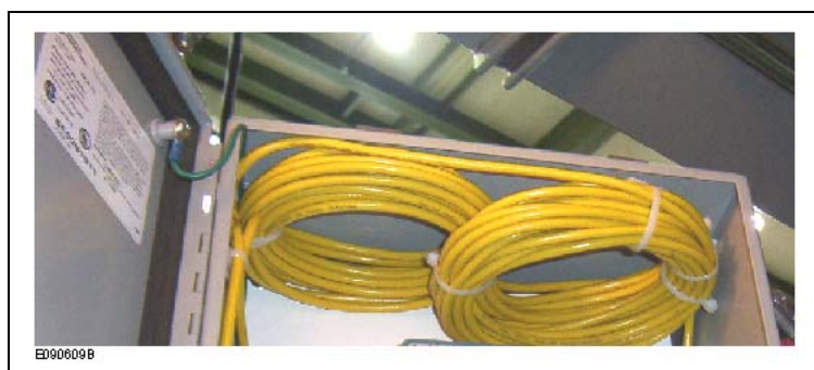
Figure 20 : Surplus cable stored inside a protection cabinet
