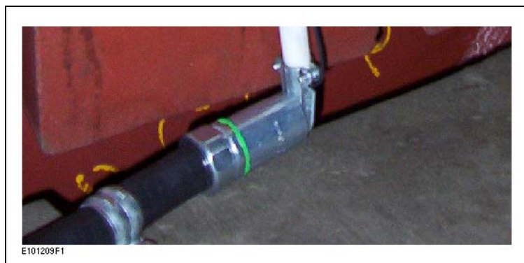
Figure 19 : Flexible conduit attached to the elbow assembly
