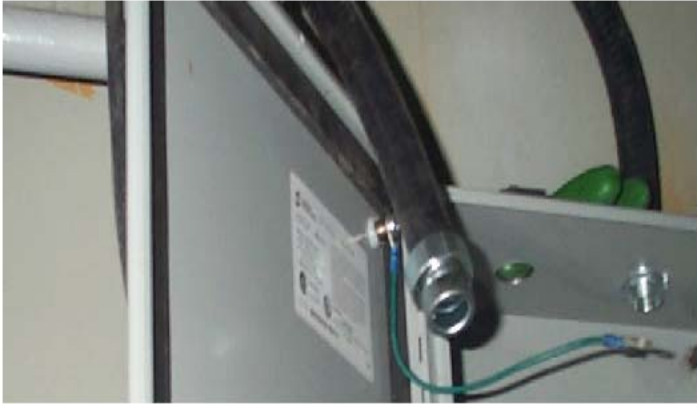
Figure 17 : Attaching flexible conduit to a protection box
