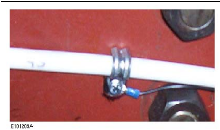
Figure 14 : Attaching the grounding wire to the structure through a cable clamp
