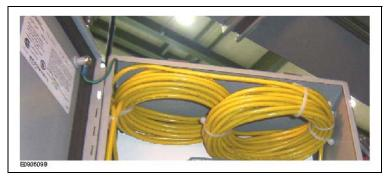
Figure 30 : Excess cable stored in enclosure
