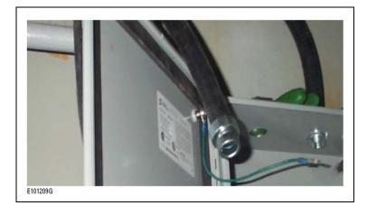
Figure 27 : Flexible conduit connection to enclosure
