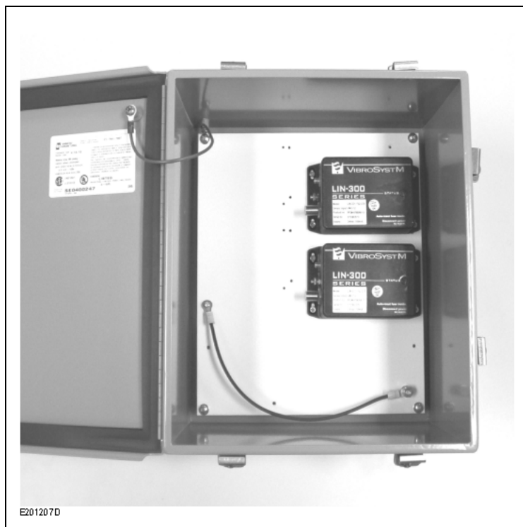
Figure 24 : Pair of LIN-300 Series modules inside a protection box
