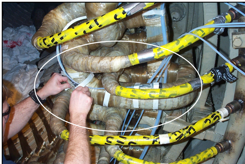
Use of adhesive tape to hold FOA accelerometers sensors FIGURE 3
