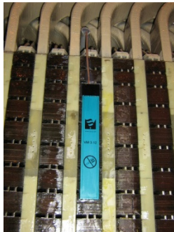
VM3.12 Air gap sensor on stator wall
