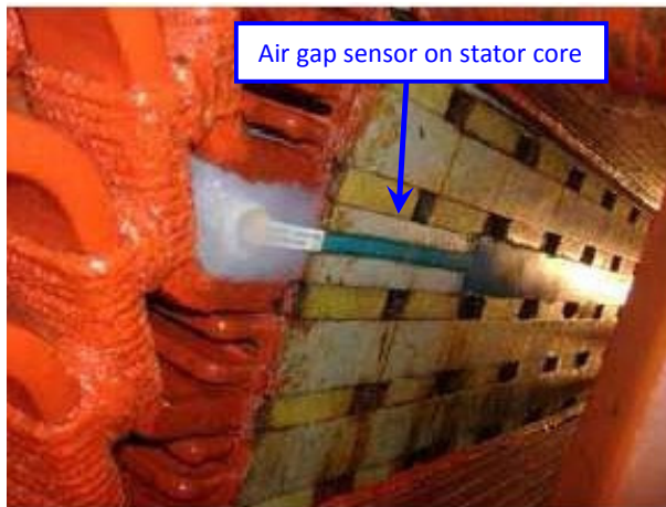
Air gap sensor glued to stator core.
