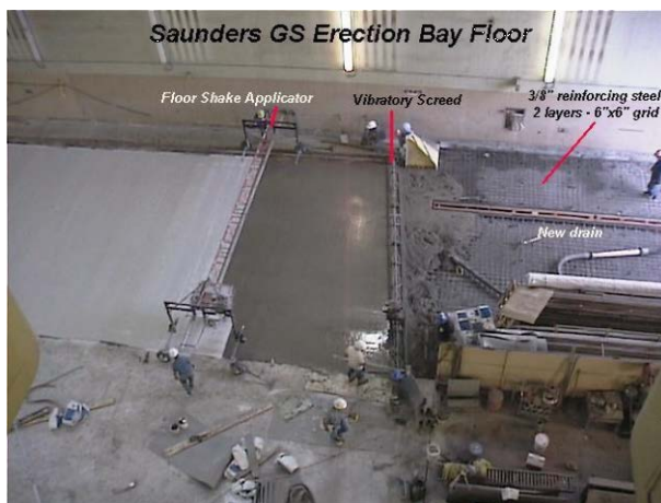
Figure 9 - Erection bay floor replacement
