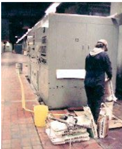
Figure 7 - Preparing to grout around a governor cabinet
