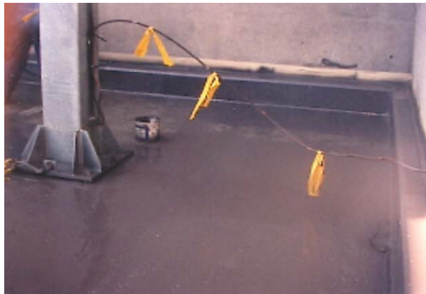
Figure 13 - Transformer bay oil containment liner
